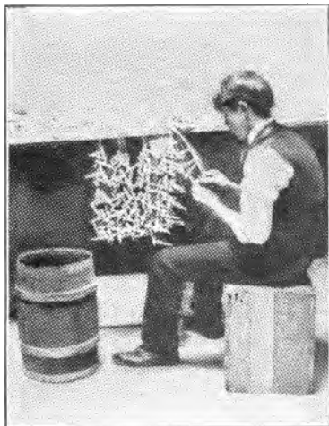
Fig. 42. Old Method of Plating Small Articles.
